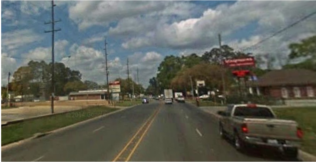
Figure 2.2. Before condition of LA 182
